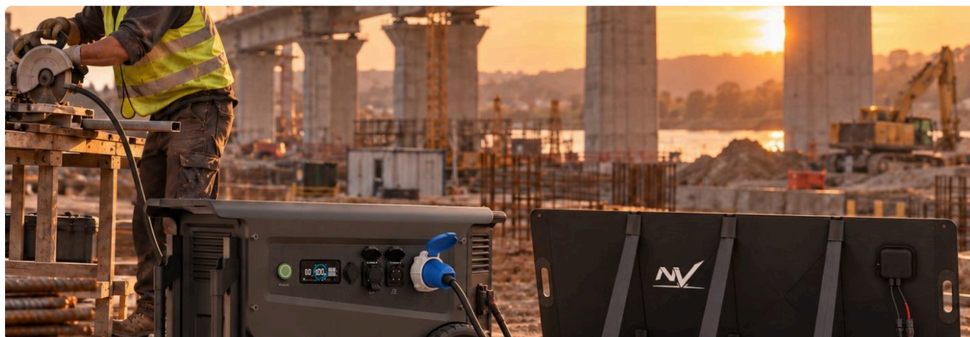
NV-S240 and NV-W50: bridge works
